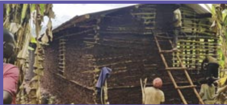
The chicken house under construction.
